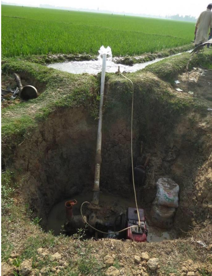
**Figure 2.27** STW installed below the ground level to pump water during the driest period
