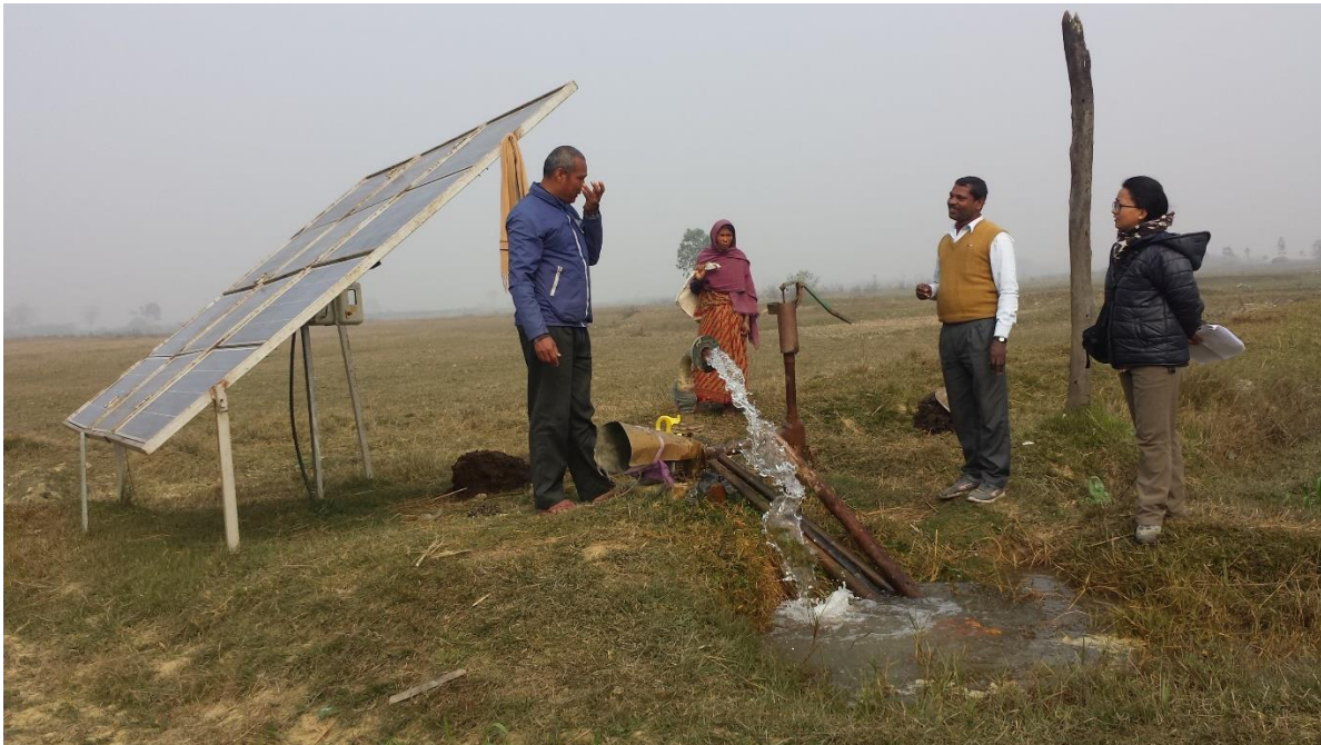
Figure 15: Solar pump installed in open area without fence, Surunga Municipality-7, Saptari
