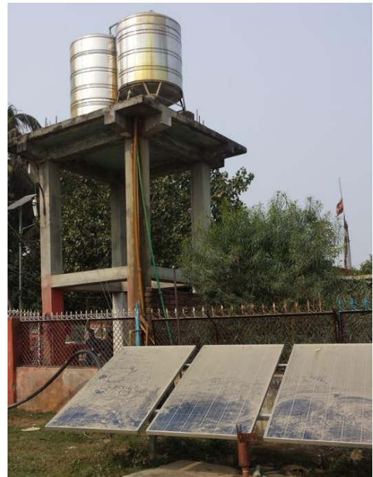
Figure 13: Solar Water Pumping System at ChhinnaMasta Temple, Saptari ( not in Function since last six months )
