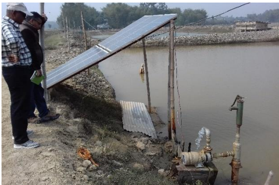
Figure 9: Solar Pumping System (900 Wp) at Fish Pond (Rupani Rural Municipality-1, Saptari)
