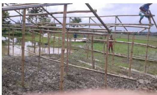
Pict.-1: Polyhouse at Uttar Chokowakheti during preparatory stage
