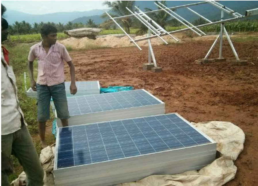
ERECTION OF SOLAR PANELS IN THE STEEL FRAME
